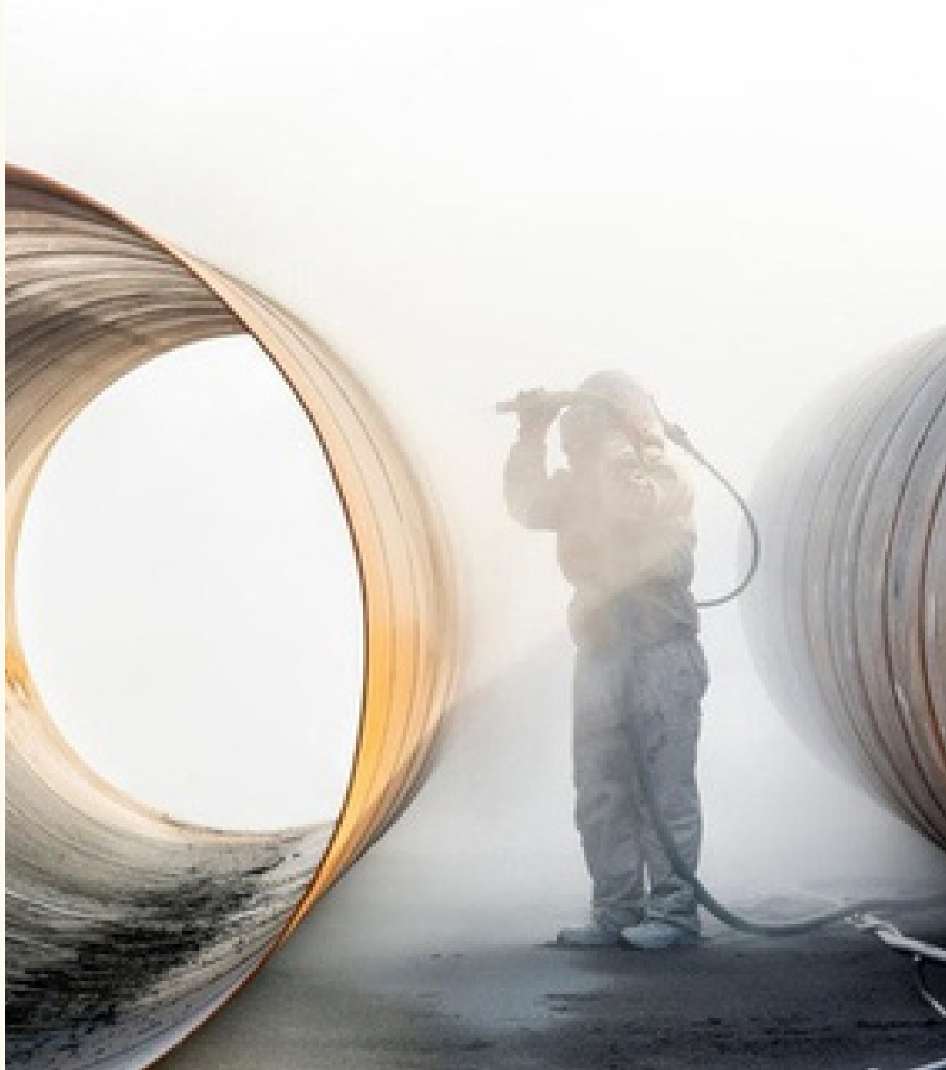
Internal & External Pipe Coating
